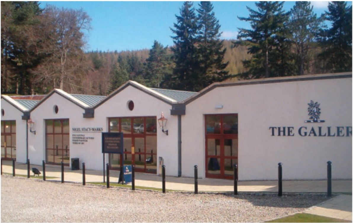
UVF films installed at House of Bruar
