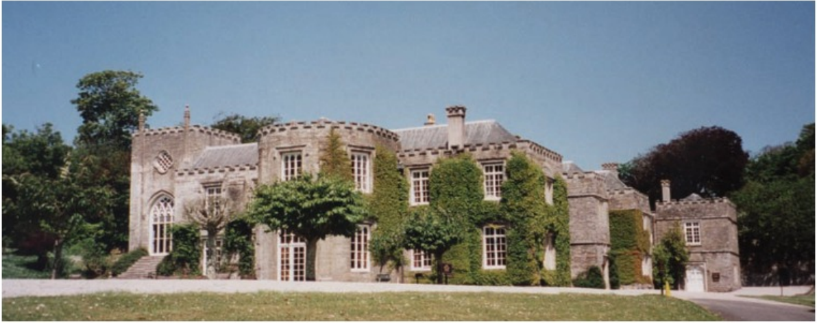
UVF films installed at Prideaux Place ( www.prideauxplace.co.uk )
