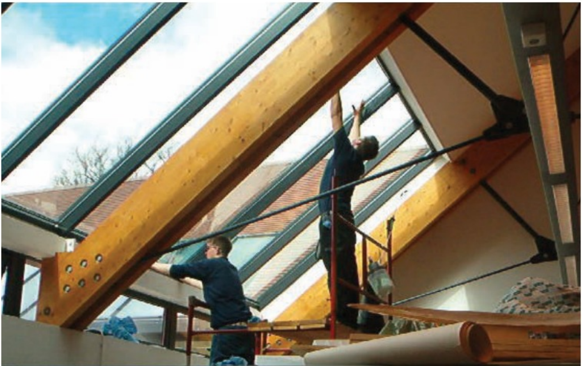
UVX films installed at University of Nottingham
