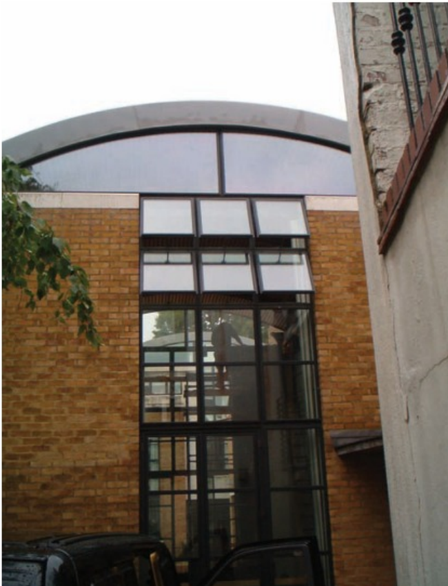
UVX films installation London (private client)
