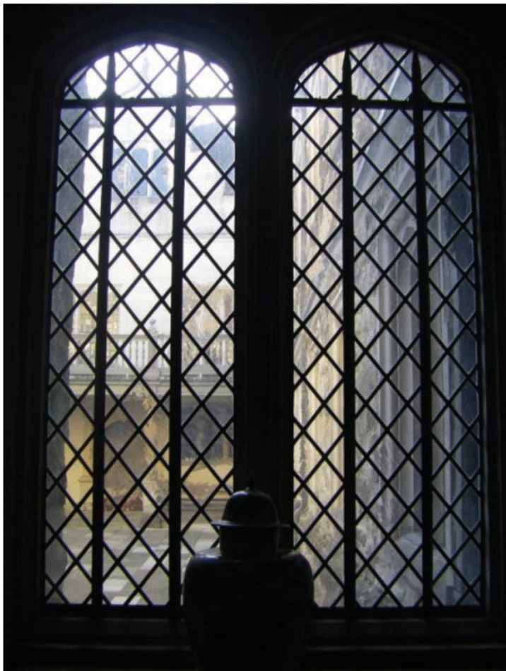
Uvista panels installed at Knole
