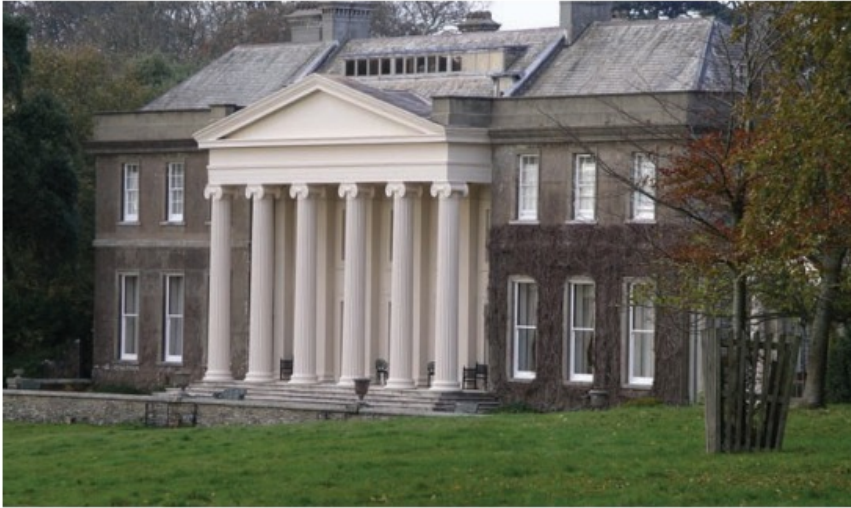
UVF films installation (private client)
