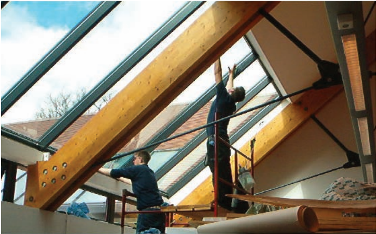
UVX films installed at University of Nottingham
