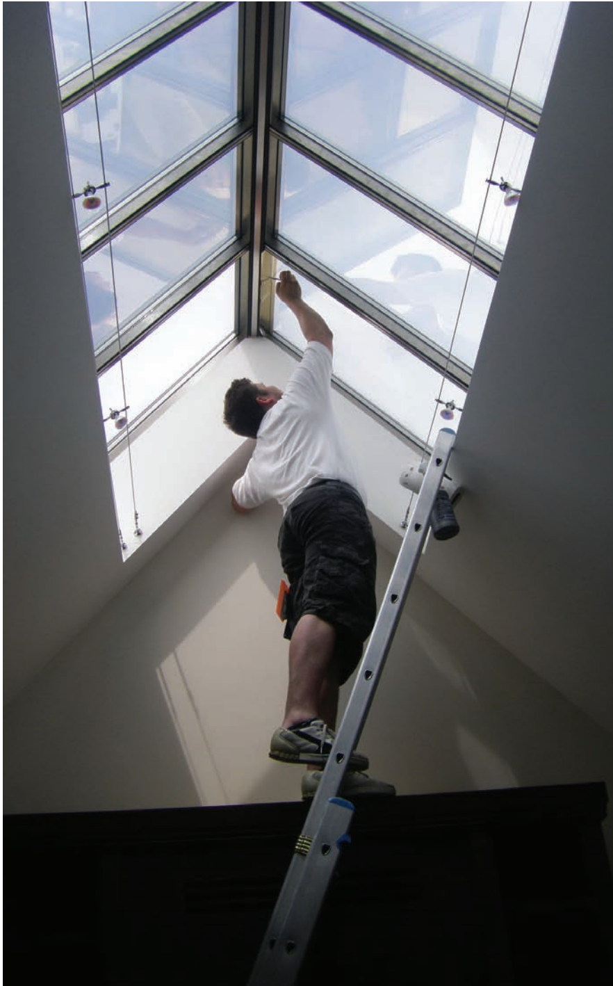
UVR films installed on an atrium (private client)
